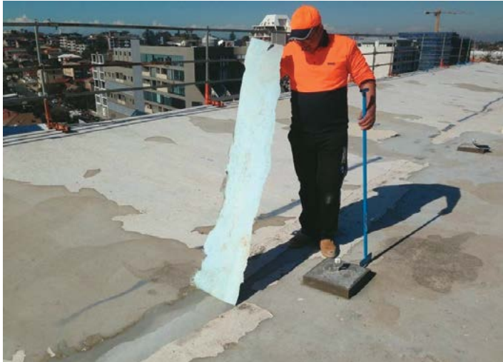
Applying waterproof membrane
